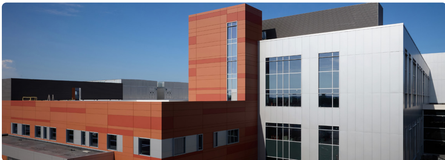
On the cover and above: MPT has invested more than $350 million to build a new, state-of-the-art hospital for the Norwood, Massachusetts community following catastrophic flooding that destroyed the former facility in 2020. The 130-bed hospital design is expected to focus on treating acute care conditions.
