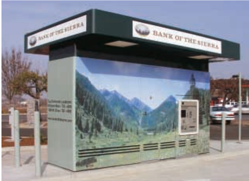
Drive-through ATM located in the parking lot of the South Valley Government Center, Henderson and Highway 65, Porterville, California.
